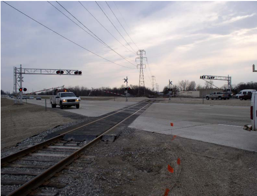
Highway Grade Crossing
