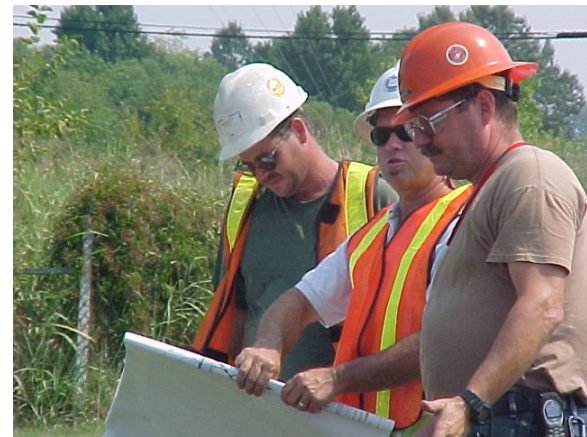
NSC FIELD ENGINEER ON SITE MEETING WITH LOCAL ROAD AUTHORITIES
